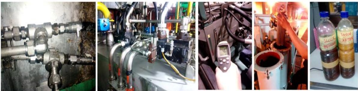
Figure 4. The function test for hydraulic cylinder.
